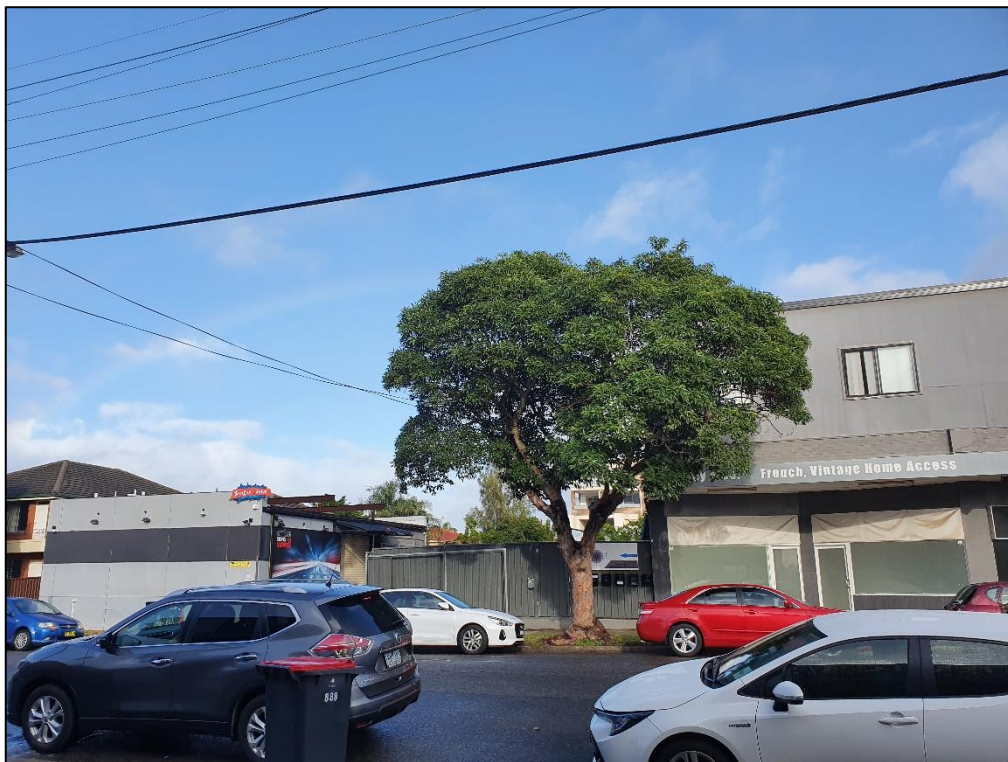
Figure 3b: Photograph of mixed use site from Flora Street
